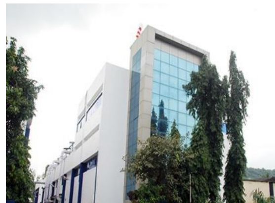
API Plant III - Patalganga
